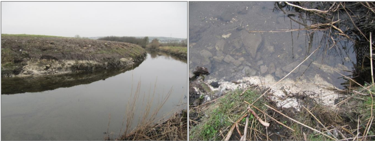
Plates 2 & 3. Marling visible along river bank at Castlegar
